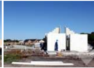
Moladi formwork re-erected on the next foundation
