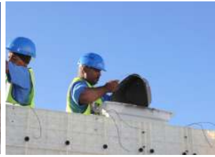
Moladi mortar mix cast in formwork cavity
