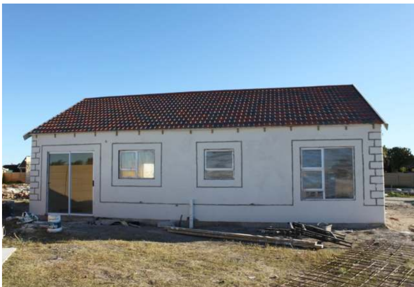
A middle-income 3 bedroom, 2 bathroom Moladi house
