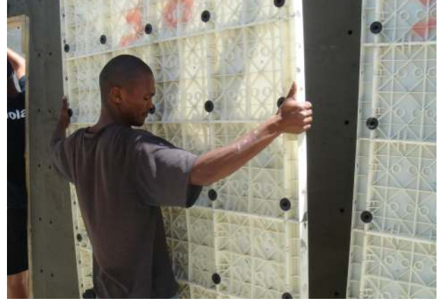
Moladi's lightweight panels allow for easy handling
