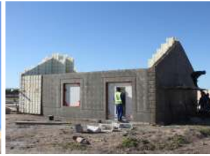
Moladi formwork panels removed
