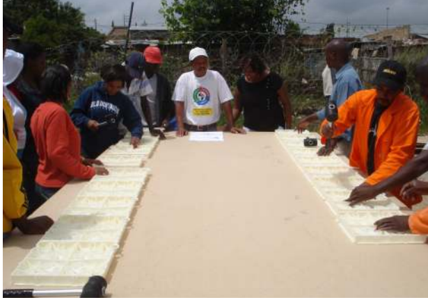
Moladi on-site training of local unskilled labourers
