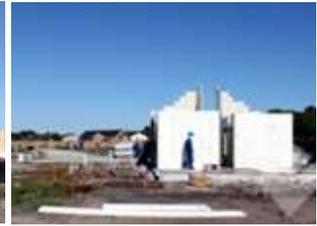
moladi formwork re-erected on the next foundation
