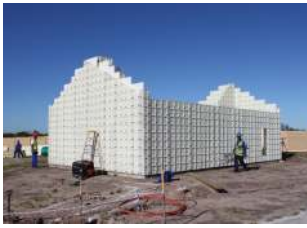
Moladi formwork panels, reinforcing steel and services erected
