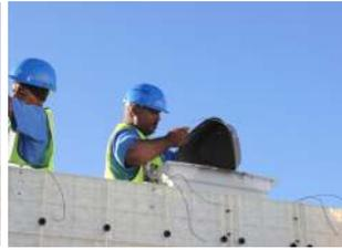
Moladi mortar mix cast in formwork cavity
