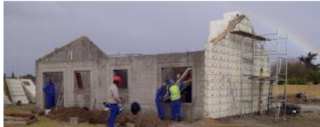
Construction Method - moladi
